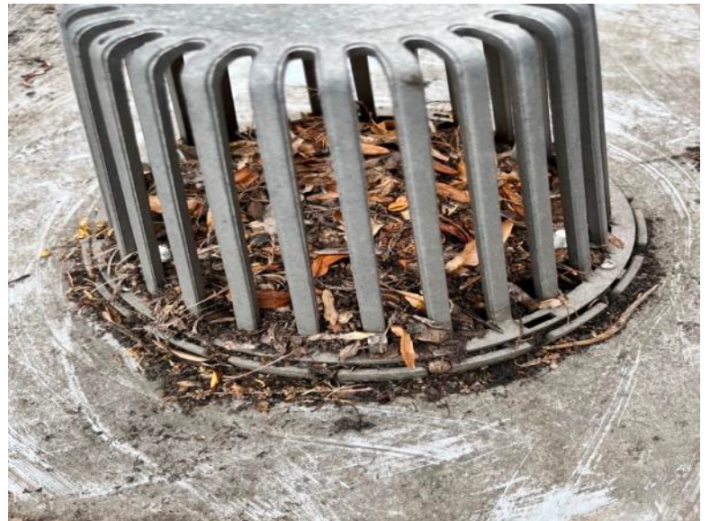
Debris covering drain opening
