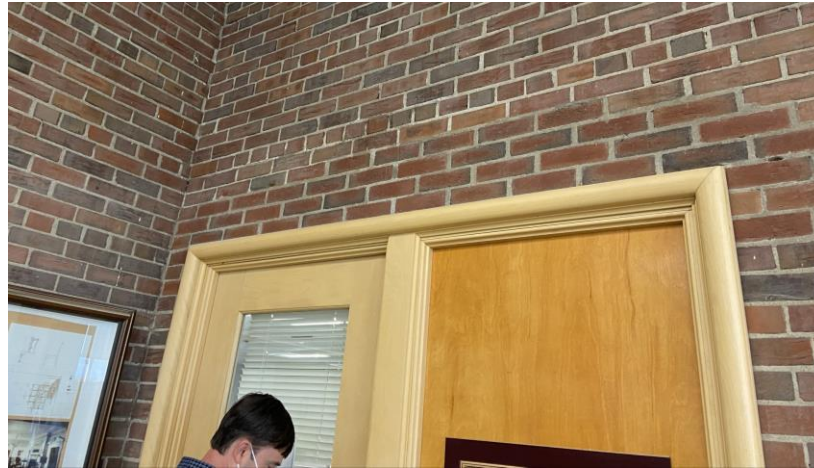
Example of unsupported masonry opening at interior door
