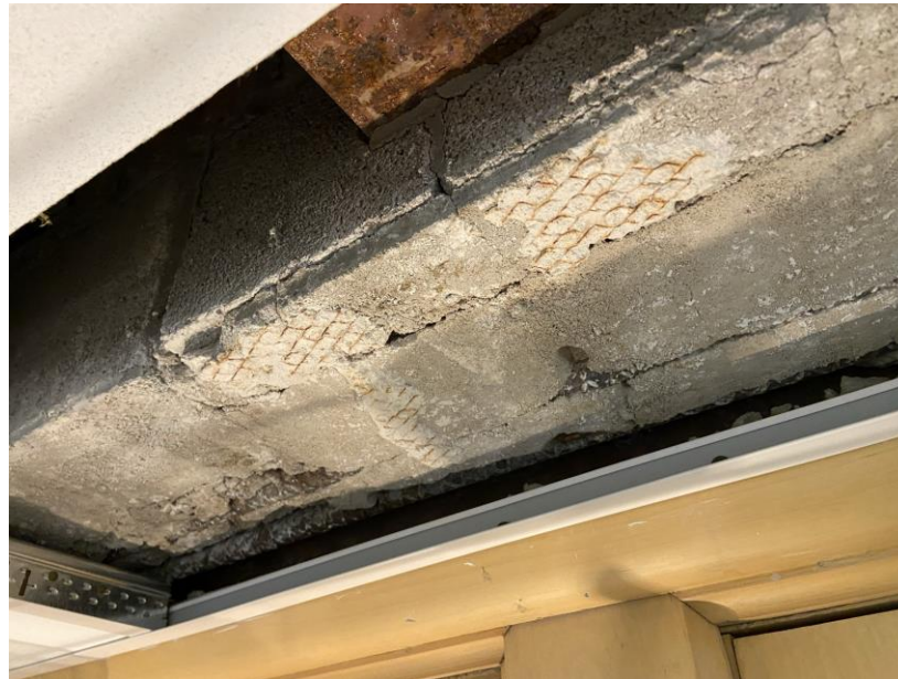
Example of unsupported masonry opening at interior door
