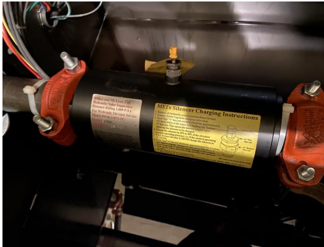
A hydraulic silencer was added as part of the modernization in/around 2011.
