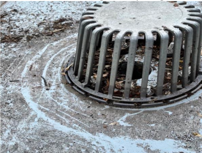
Debris covering drain opening
