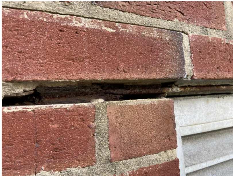
Section loss at steel lintel supporting openings over exterior louvers
