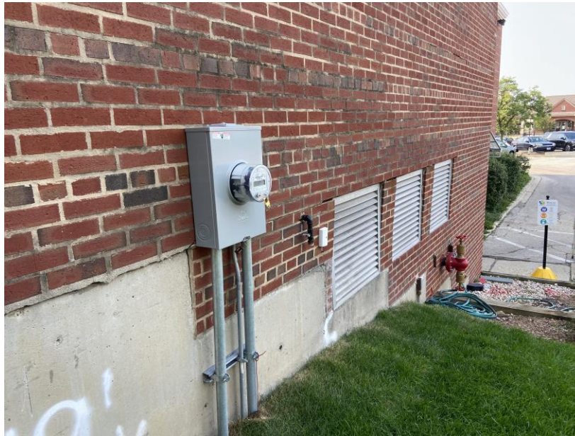
Exterior wall - discoloration and movement/out-of-plane masonry visible
