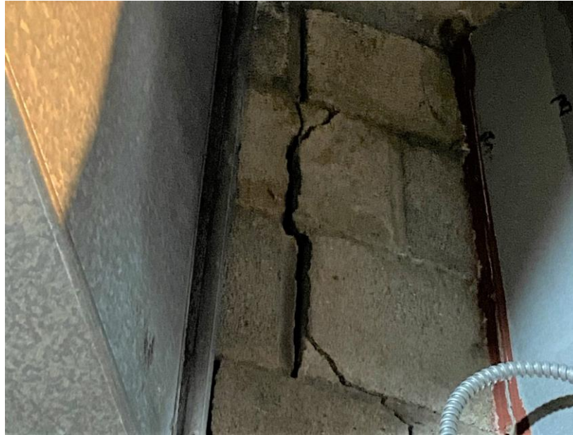
Cracks in concrete masonry at interior, between exterior louvers pictured above.
