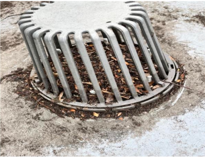
Debris covering drain opening
