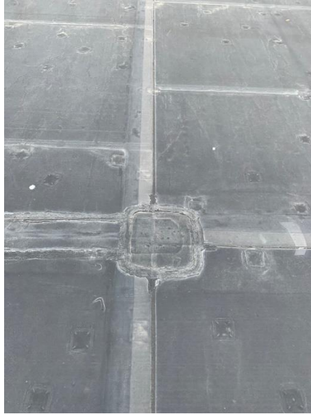
Map # 9 Overview of Roof Field seams checked
