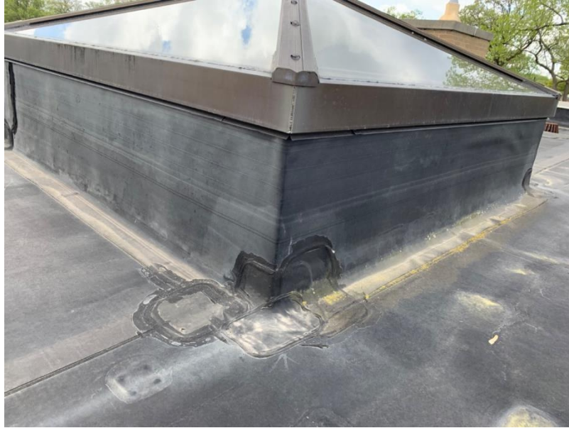
Map # 5 Overview of Roof Skylights checked
