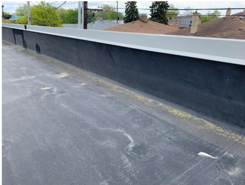
Map # 8 Overview of Roof Wall flashings inspected
