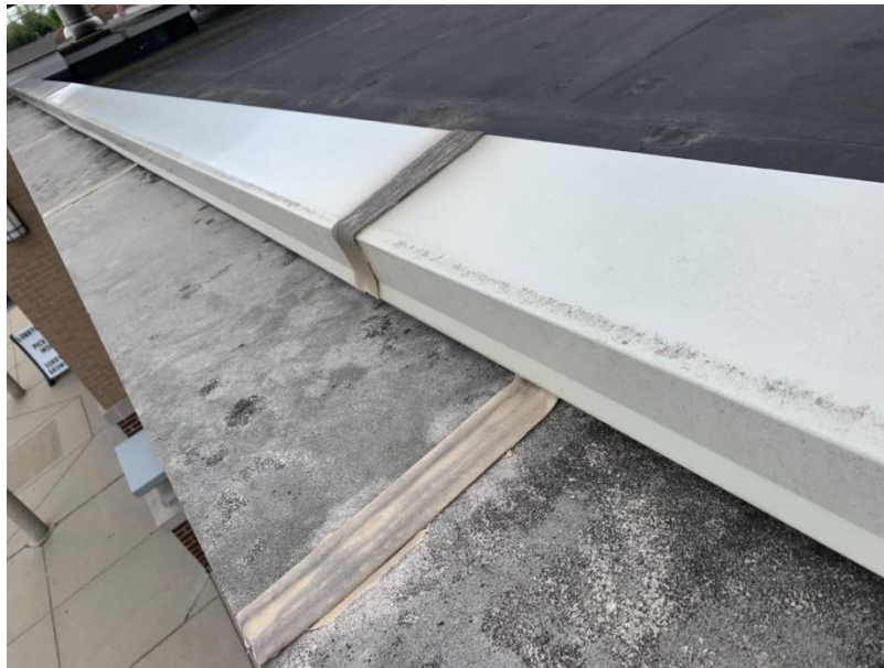
Map # 4 Overview of Roof Coping caps checked
